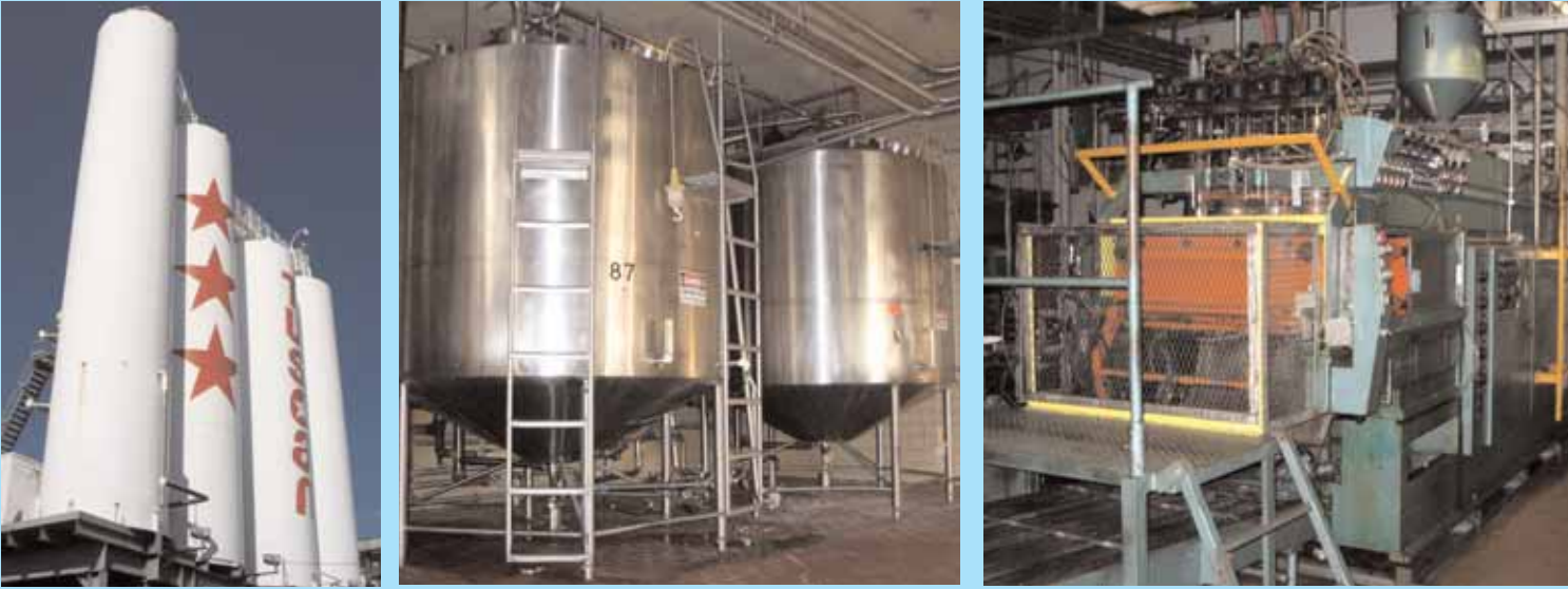
(16) S/S SILOS TO 60,000 GAL. - (15) S/S PROCESSORS - (5) UNILOY BLOW MOLD LINES
