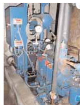
Case Stack Washer - Vilter Freon Compressor - (2) Sullair Air Compressors
