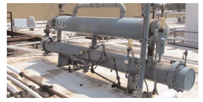
Left: (3) BAC Evaporative Condensers Below: RVS Shell & Tube Ammonia Chiller
