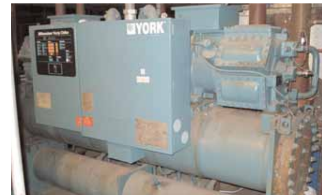
York Packaged Chiller and BAC Perma Cold Evaporative Condenser
