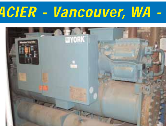
York Packaged Chiller and BAC Perma Cold Evaporative Condenser
