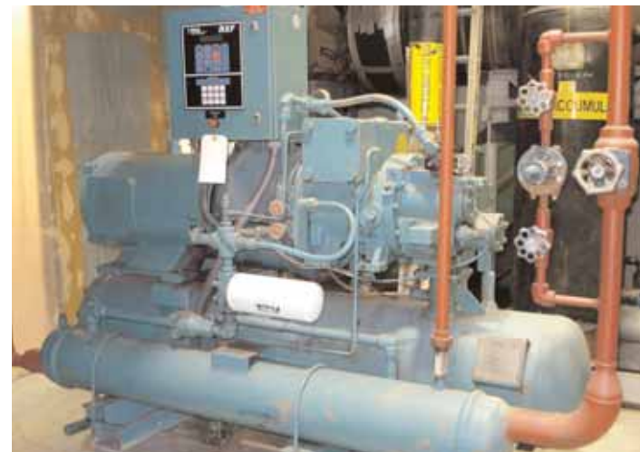
(2) Frick 125 hp Models RXF50 and RXB50 Screw Ammonia Compressors
