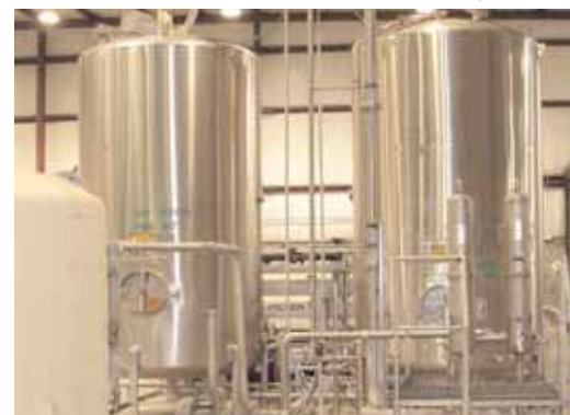
1999 US Filter & 1996 Osmonics R/O Systems
