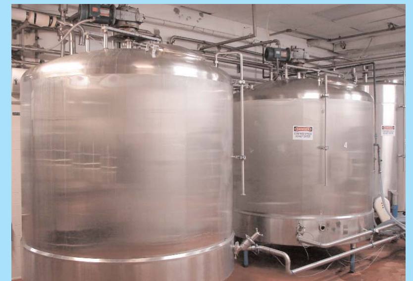
(5) Cherry Burrell Dome-Top, Dish Bottom 1,500 Gal. Tanks
