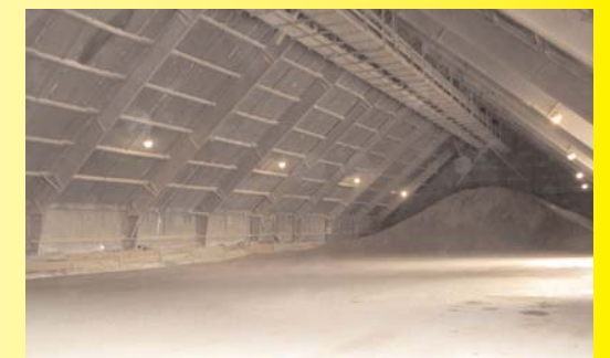
Structural Steel: I-Beams, Angles, More
