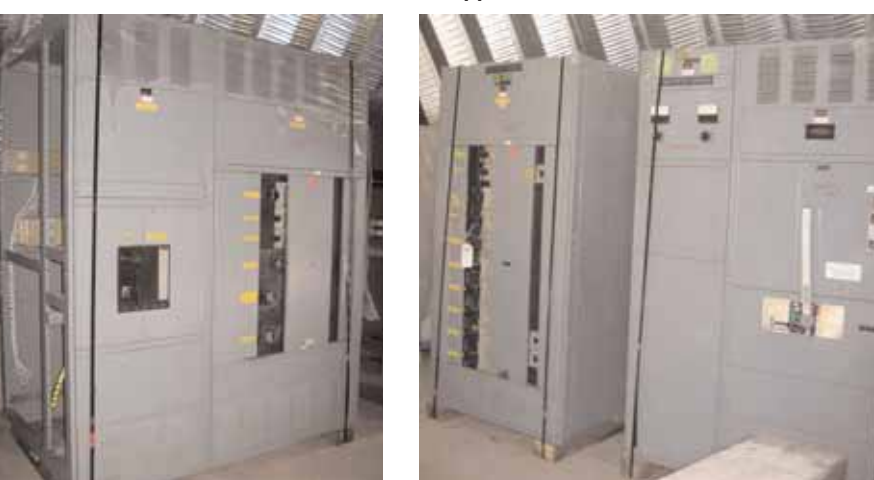
Large Selection Allen Bradley, Square D & GE Disconnects & Motor Control Centers
