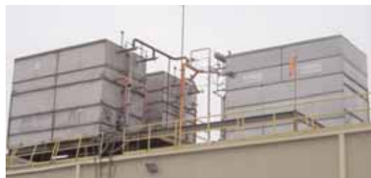
Evapco & BAC Evaporative Condensers
