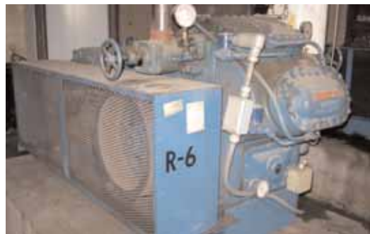
(6) Vilter Ammonia Compressors up to 400 hp
