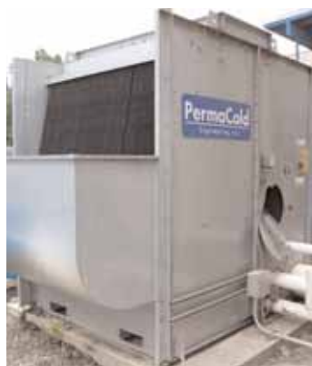
PermaCold Cooling Tower - Evapco Evaporative Condenser
