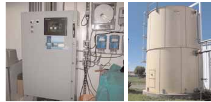
2004 DAF Waste Treatment System Controls & Tank
