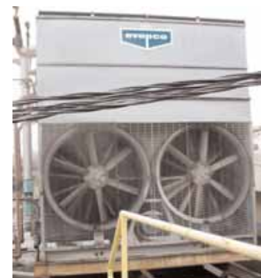
PermaCold Cooling Tower - Evapco Evaporative Condenser
