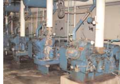
Evapco Condenser, Delta Cooling Tower, CO 2 Tank - (7) Vilter Ammonia Comp. to 150 hp
