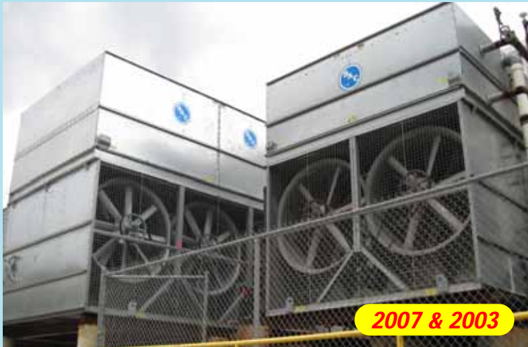
2007 & 2003 BAC Evaporative Condensers
